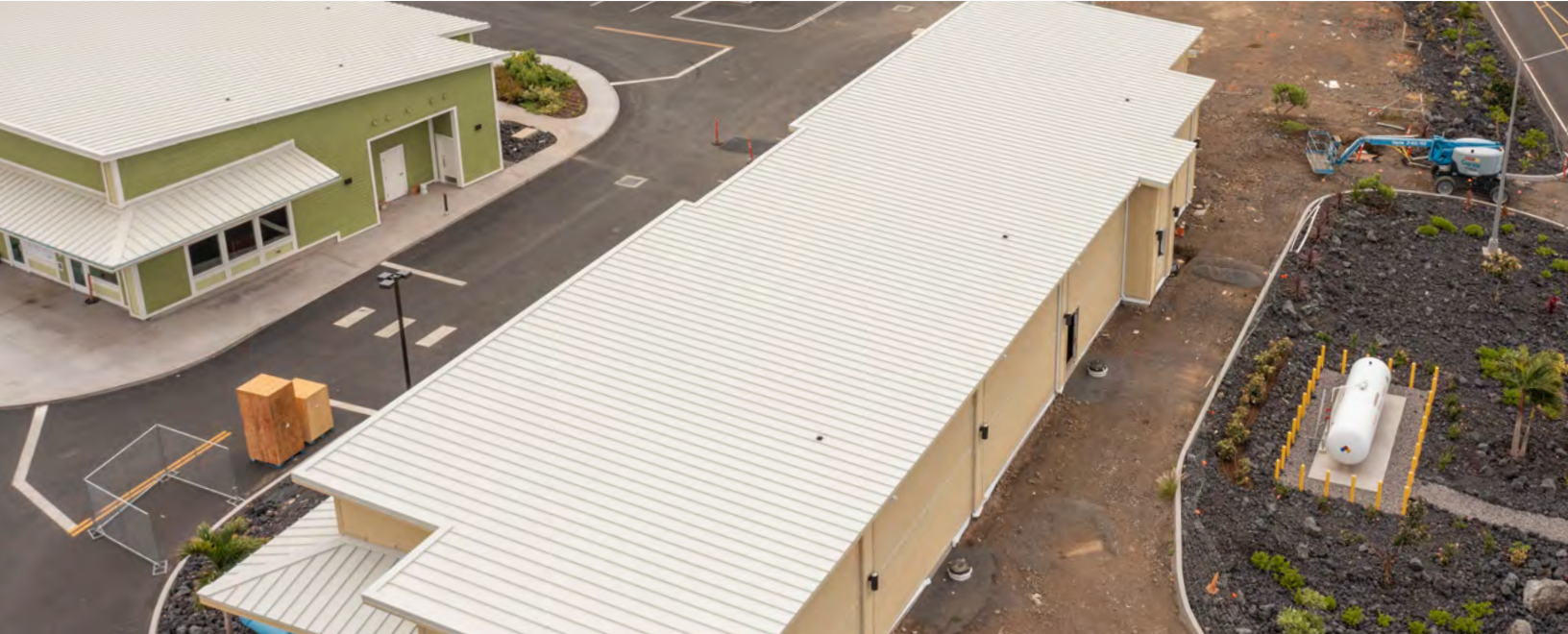
Building J (Kohala Coffee Co., Pudjee Panda & Coco Cantina) shell construction is ongoing. Walls, building trusses and roofing have been installed. Pudjee Panda & Kohala Coffee, & Coco Cantina tenant improvement plans are under review by county. Siding installation is on going.
